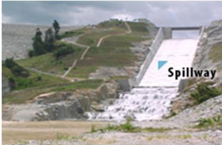
Fig. 13.2. Chute spillway.
