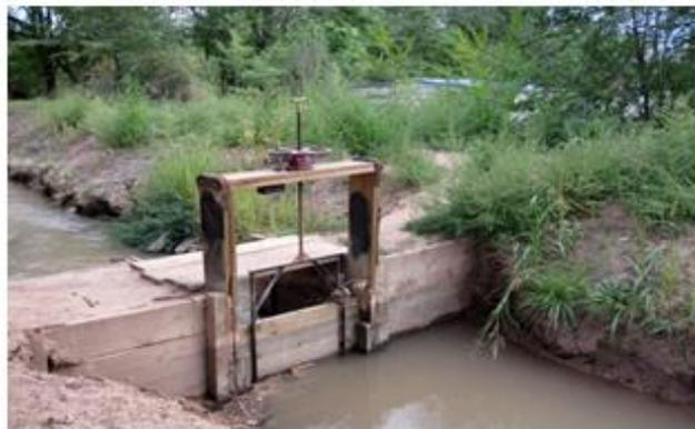
Fig. 14.1. Canal check gates.
