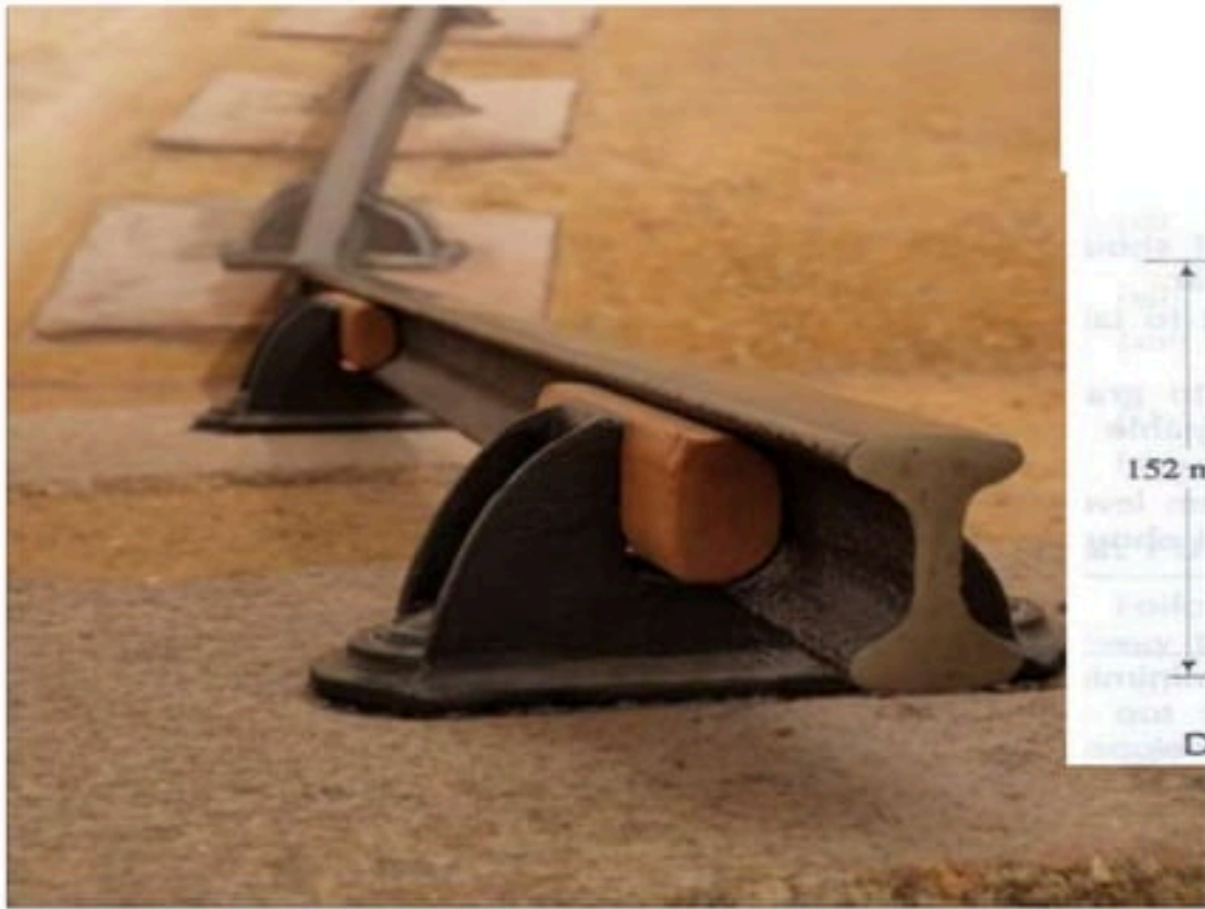
Fig. 1 Double headed rail
