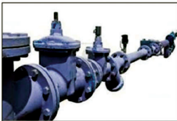
Fig. 5.27: Flanged joints
